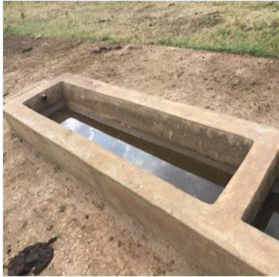
c) Water trough on site
